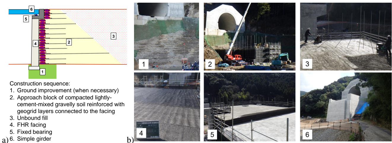
Figure 6. GRS bridge abutment: a) structure; and b) construction on a slope at Sugamuta viaduct.
