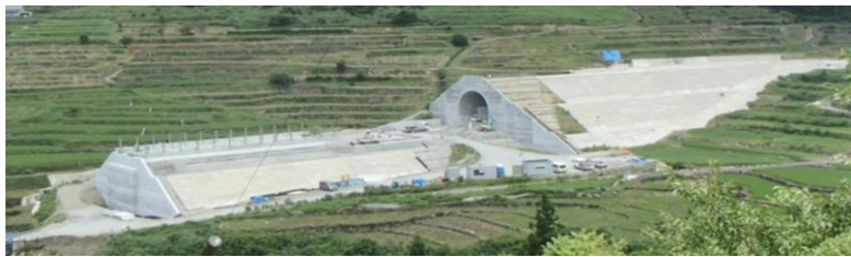
Figure 13. GRS tunnel entrance protection and GRS bridge abutment, Tawarazaka, Nagasaki Pref. side.
