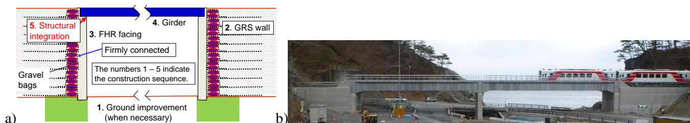
Figure 7. GRS integral bridge: a) structure & construction; and b) Haipesawa bridge, 60 m-long, Sanriku Railway.
